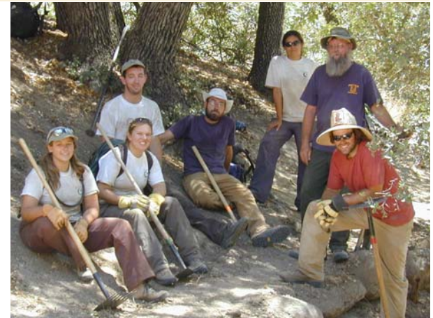
The SCA crew takes a break from trail work.
