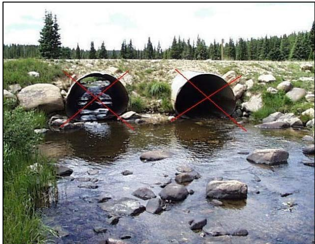
Two failing arch pipes were replaced with one bottomless arch. Photos by Greg Eaglin.
