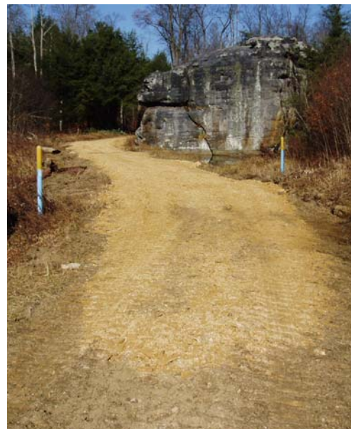
Before and after road reconstruction. Photo courtesy Allegheny National Forest.
