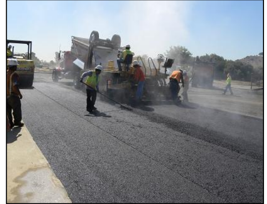
Typical asphalt job. Photo courtesy SDTDC
