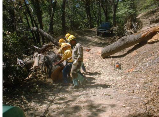
Volunteers clear a Forest road. Photo courtesy San Bernardino National Forest.
