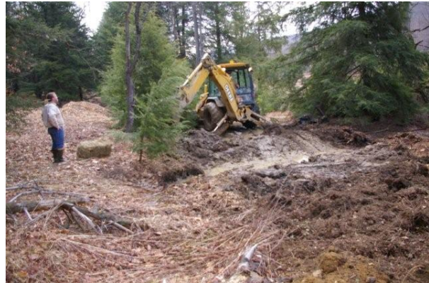
Decommissioning a roadbed adjacent to the North Country Connector.
