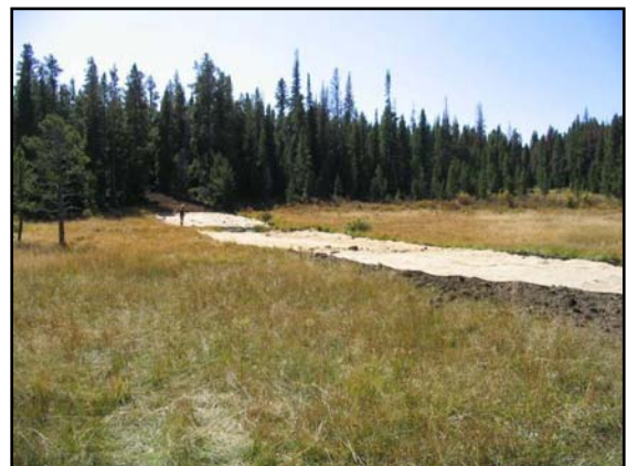
Wetland crossing fill, before and after removal. Photo credits: Top: Dave Gloss. Bottom: Laura Jungst
